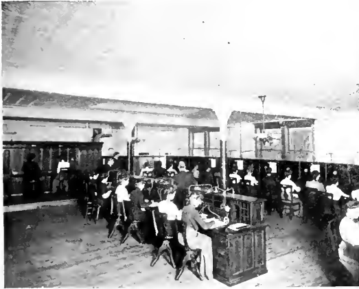
FIG. 3.—TOLL LINE OPERATING ROOM.
